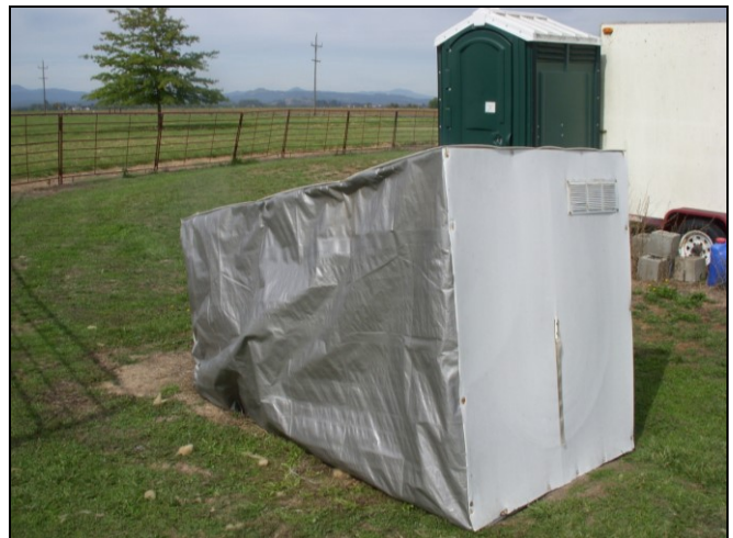
Mower shed in need of repair
