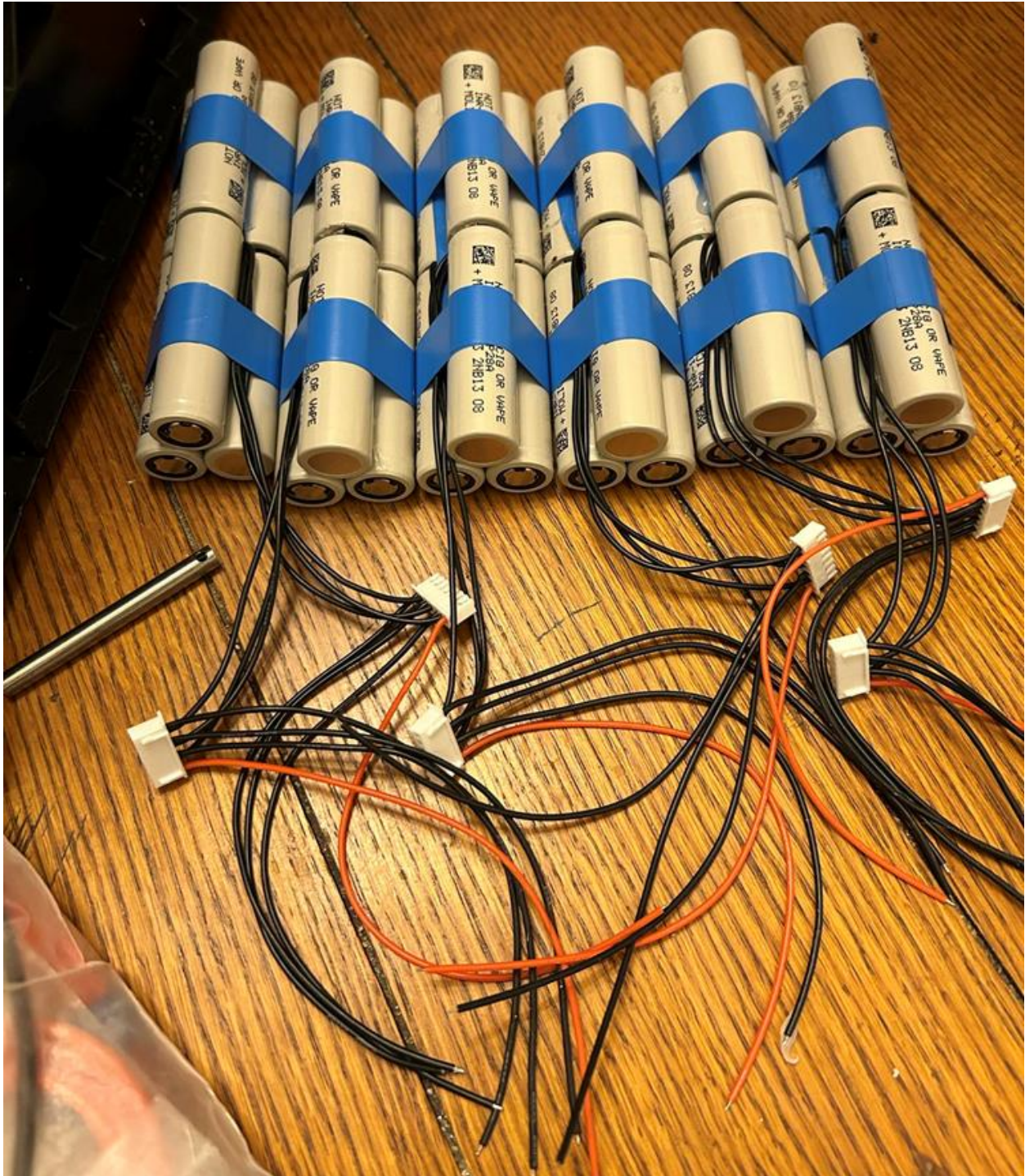
Li-Ion batteries before applying shrink wrap (Photo by Dane Martin)
