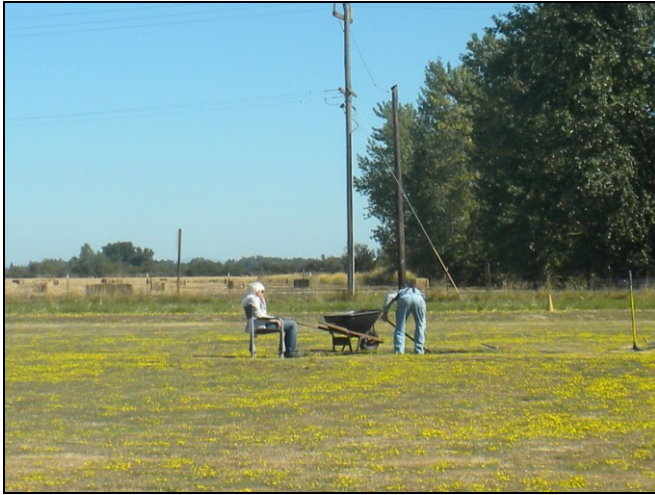
Gary re-working circle center pad
