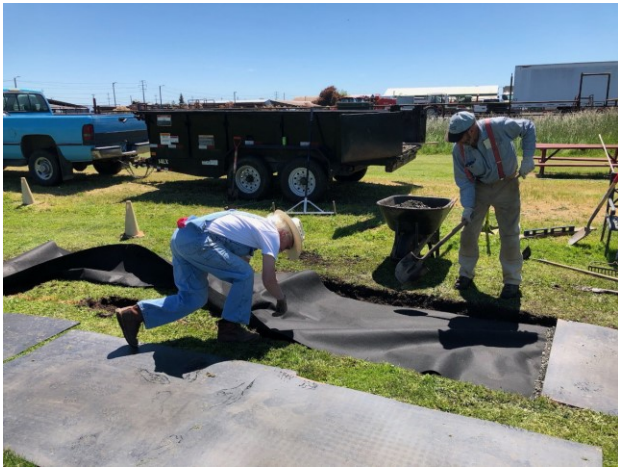
Gary and Dave dug out sod, laid in fabric.
