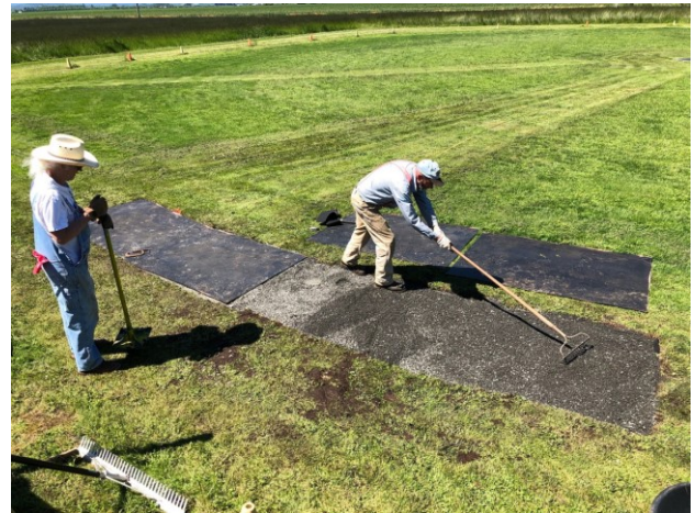
Cover fabric with gravel and smooth it out.
