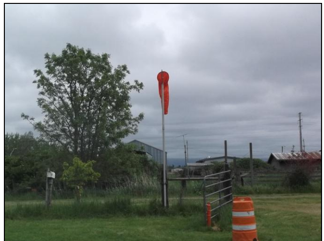
New windsock installed
